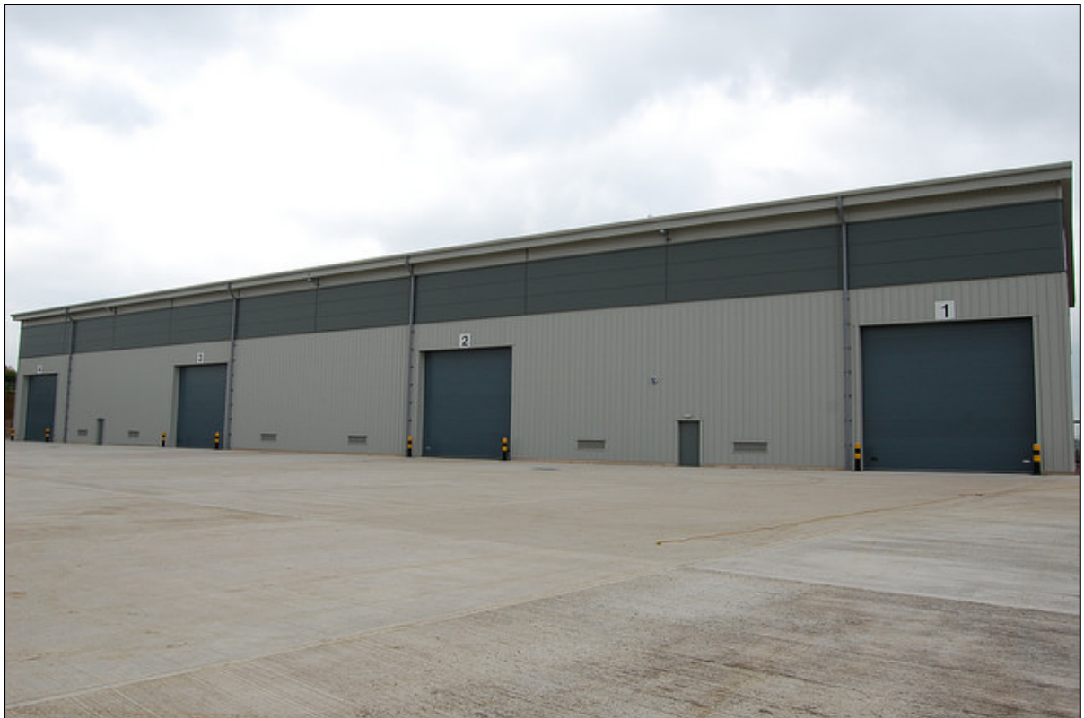
Photo 1 Lower House Farm Waste Transfer Station (licensed to hold 80, 000 tonnes per year)
